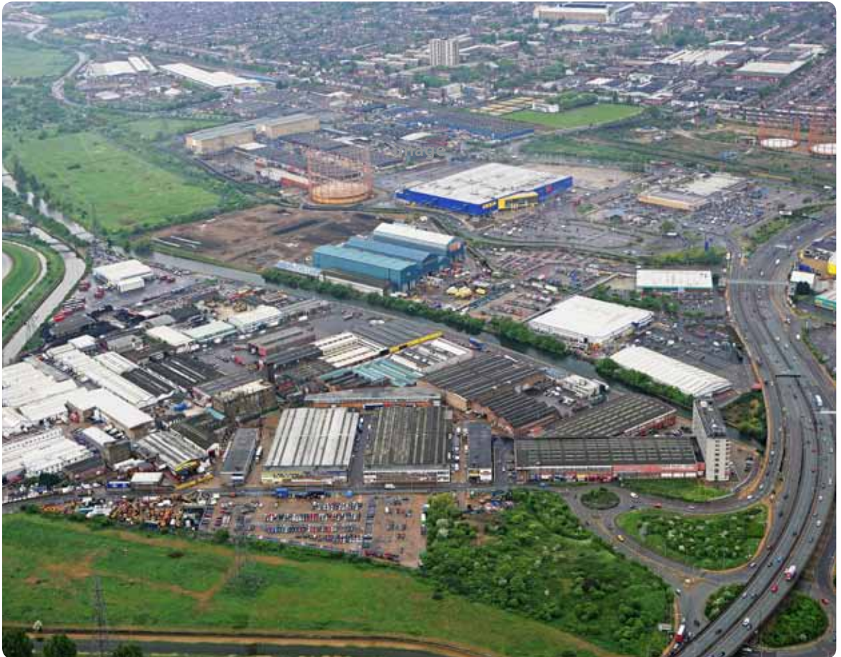
Harbet Road Industrial Estate and Meridian Water
