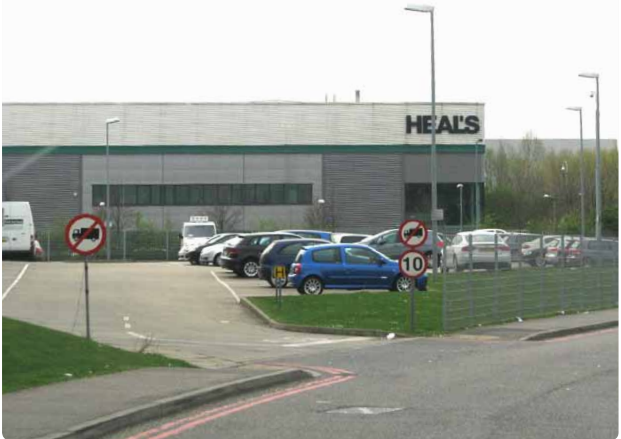
Heal's Distribution Centre, Aztec 406 Industrial Estate
